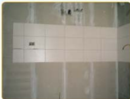
8-Putting tiles on sink places
