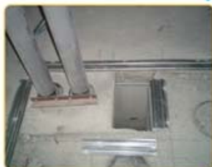
2- Channel installation
