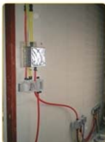
8- Electric Box Installation
