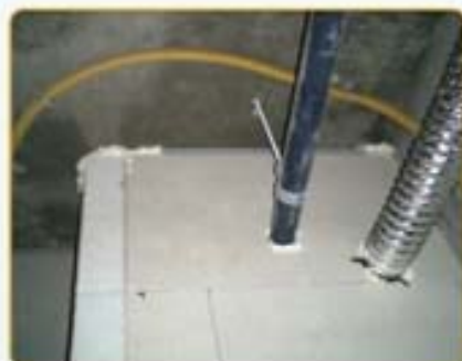
4- Panel installation finishing
