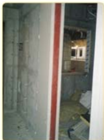
10- Housing wall back side Instalian
