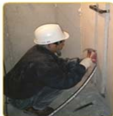
6- Facility pipe landfill
